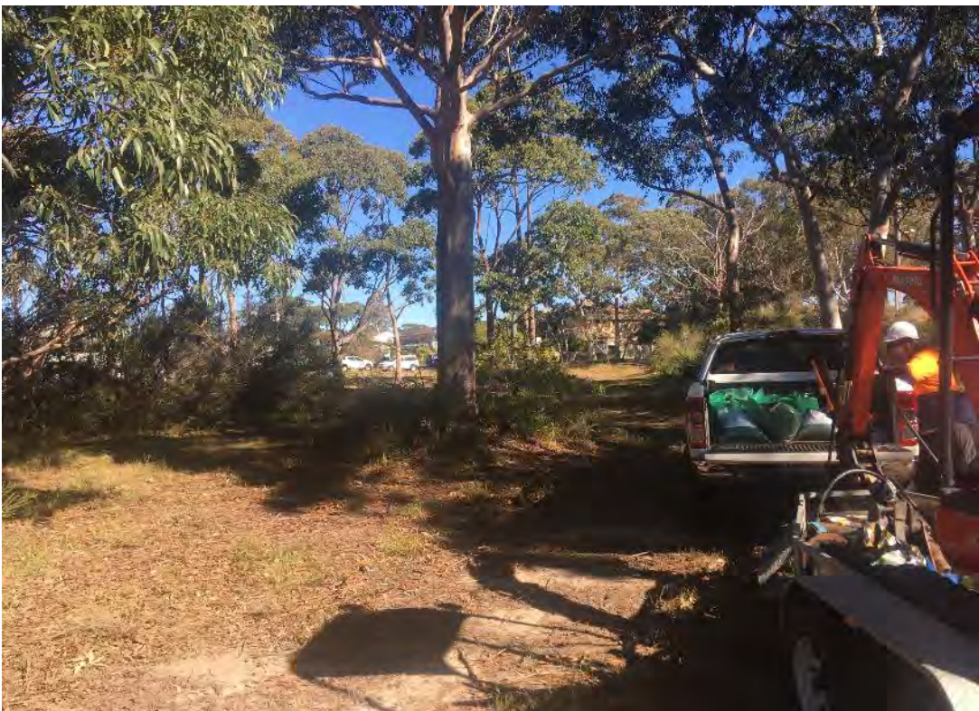
Photograph 12: South-western portion of the site, looking south-west towards Monarch Place.
